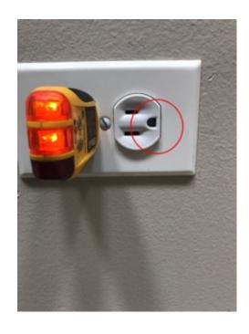
**Condition: GFCI broke** - The Ground Fault Current Interrupter is broken. Its safety capabilities are therefore eliminated. Replacement is needed.
