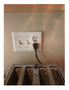
**Three-prong** - Ground plug is broken off in receptacle therefore not allowing a grounded plug to be plugged in. I suggest a certified electrician evaluate further.
